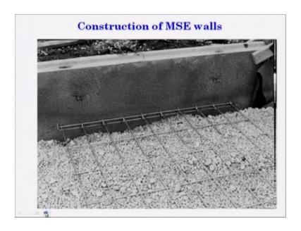
Now, this is this is the things w which to have discuss this reinforcement. Once you place a layer of soil, once you place a layer of soil along with this layer of soil, you can provide reinforce middle layer this is your enforcement layer in the form of or greet.
