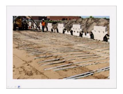
In the case of mess these are all single reinforcement single reinforcement, in terms of flex small thin plates it has been placed with this spacing it has been placed in the layer f soil layer over this.
