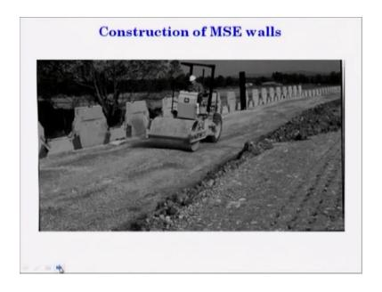
Then you can do the roller in compact it by means a by rollering it ten's that layer is over, then again you place another layer of reinforcement, then wheel a soil, then compact it. So, this construction will be layer by layer; that means, it is consisting of a
