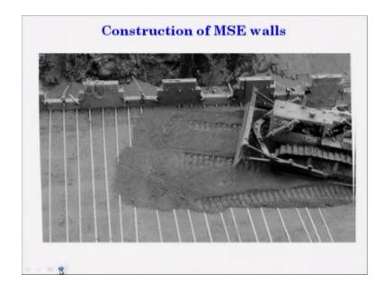
Then once this reinforcement has been placed above this reinforcement, you place again you start construction of another layer of soil must I am talking about how the construction has been done another layer of soil must you can place it over the once the reinforcement has been placed.
