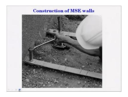
Then this reinforcement has been properly tide, and fix in the soil mass you see earlier enforcement.
