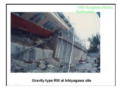
If you look at here gravity type of retaining wall; it happened in 1995 earthquake, Nanbu earthquake. This is your gravity retaining wall, this retaining wall is gravity retaining wall, the damage has been made, it has been taken from that side, how the damage is there, because of earthquake.
