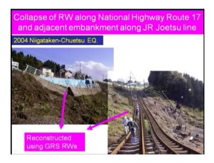
Then collapse of retaining wall along National Highway Route seventeen. If you look at here, reconstructed during ah particularly using GRS retaining wall. GRS retaining wall, how the construction has been going on. This is the first one is your means collapse of your retaining wall. And this is by using your reinforced earth how this construction process is going on.
