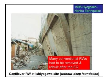
Now second one is your cantilever retaining wall. If you look at here, this is your cantilever retaining wall, this damage because of your nineteen ninety five ah Nanbu earthquake. Then this cantilever retaining wall is without any deep foundation.
