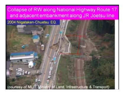
Second is your collapse of retaining wall along National Highway Route seventeen and adjacent embankment along Joestu line. It is said 2004 Niigataken earthquake. If you look at here, it is in this particularly, this area is your 56 kilometer and sorry 56 meter. It has been damaged because of your earthquake.
