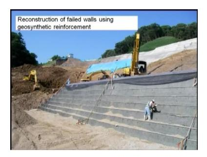
Reconstruction of failed walls using geosynthetic reinforcement. If you look at here, reconstruction of failed wall using geosynthetic reinforcement, these are all your geosynthetic by using geosynthetic reinforcement. Geosynthetic reinforcement if you look at here, geosynthetic reinforcement, there is a reconstruction of this failed walls.
