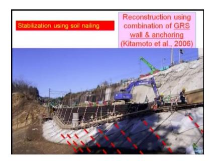
Then reconstruction using combination of geosynthetic reinforced retaining structures wall and anchoring. If you look at here, these are all your anchoring. Anchoring has been made, here this point if you look at this, this is a point of your anchor, anchoring has been made, this is a point of your anchoring. Along with your geosynthetic stabilization also soil nail, these are all called anchoring by means of soil nailing.
