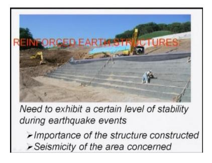
Now reinforced earth structure; it is particularly this why there is reinforcement required particularly earth structures, to exhibit a certain level of stability against your earthquake events that means how importance of the structure and particularly that area of what is the seismicity of that area concerned, that will also taken into consideration.
