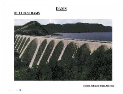
Now, look at this examples buttress dam first one buttress dam, if you look at their buttress dam upstream side buttress dam, if you look at here in quebec one cases of buttress dam.
