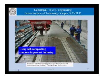
This picture here, shows the use of self-compacting concrete in the precast industry, there is concrete members, as can be seen here are being cast using concrete with very little intervention manually and these people here are just doing some preliminary or some simple leveling operations. So, that is another application of self-compacting concrete or how self-compacting concrete mix the life easier as far as the concrete engineer is concerned.
