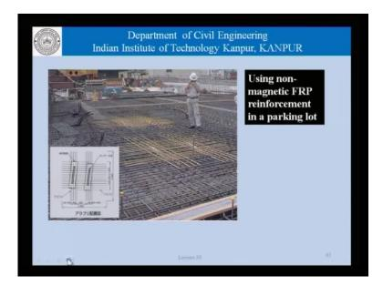
This is another application of FRP where its nonmagnetic properties are being used in a lot. Because there are some devices embedded in the slabs, which will help detect the presence of a car, when it is parked. And, if there is a normal steel reinforcement that may not be possible; and therefore, FRP may be used in at least certain places where those senses are placed.
