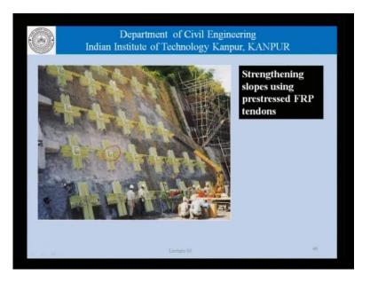
Yet another example of using FRP's in concrete construction or civil engineering construction is in strengthening slopes using pre-stress FRP tendence as I shown here.
