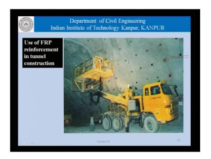
Here we are using CFRM in a tunnel construction. So, we can see that there are there is a net which has been placed using these bolts to hold a lining which is going to be applied on the tunnel.
