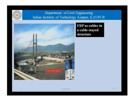
These cables are FRP cables in a cable-stayed bridge.
