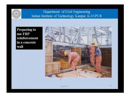
Similarly, here we are looking at FRP reinforcement being placed, which again is a grid as shown here; for the reinforcement in a concrete wall. In this case, we are using FRP as cables.
