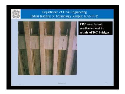
This is another interesting example of using FRP as external reinforcement in the repair of RC bridges or reinforce concrete bridges. Let me explain what external reinforcement in repair work is.
