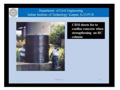
This is another example where CFRM sheets have been used for a strengthening of RC columns. We can see that as far as the concrete here, this is concrete; we can see that the concrete here in the column has now been wrapped using this FRP sheets. Now, how this helps as far as strengthening is concerned is by the following action.
