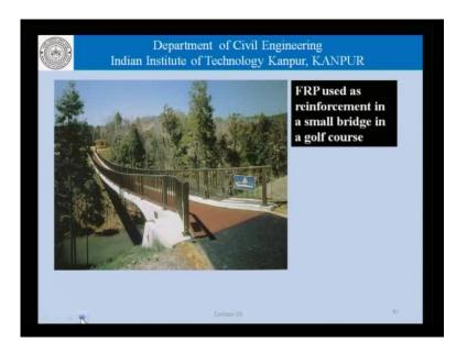
This picture shows the fiber reinforce plastics being used as a reinforcement in a small bridge, in a golf course.
