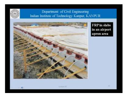
Another example is shown here; where we are trying to use FRP in the reinforcement of slabs, in the airport apron area.
