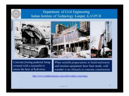
This picture here for example, shows a enclosed structure which has been erected, in order to protect this concrete. Similarly, as far as panels are concerned, we could see the covering of membranes. As far as this picture is concerned, it is just an application of curing compounds being spread on concrete to service effective sealants.
