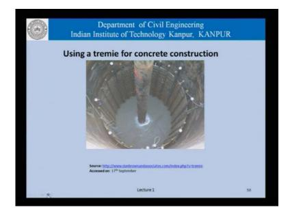
This slide shows construction of concrete with the tremie, now in this case concrete is being deposited at depth possibly under the water using a tremie. Now, the concrete is been dropped all the length of this pipe and it is ensured or it needs to be ensure that the pipe is always embedded in the concrete as more and more concrete is dumped.
