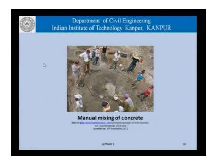
So, that you can see that water is been dumped into this larger pile here, where all the ingredients have been put together and a kind of mixing process is as that will be completed in this it will be different.
