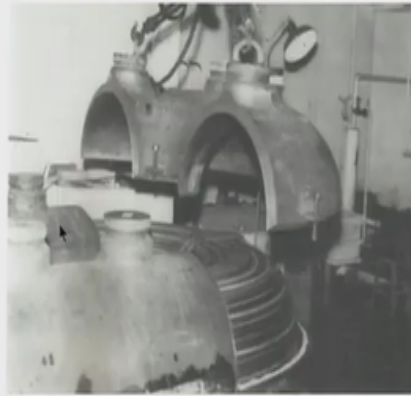
A photograph of steam generator of torus section (Courtesy-Babcock & Wilcox Co.)
