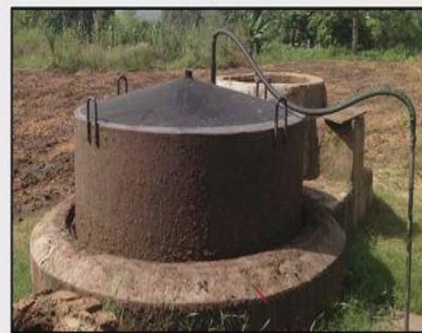
A floating drum type biogas digester in Mangalore, Karnataka, India
