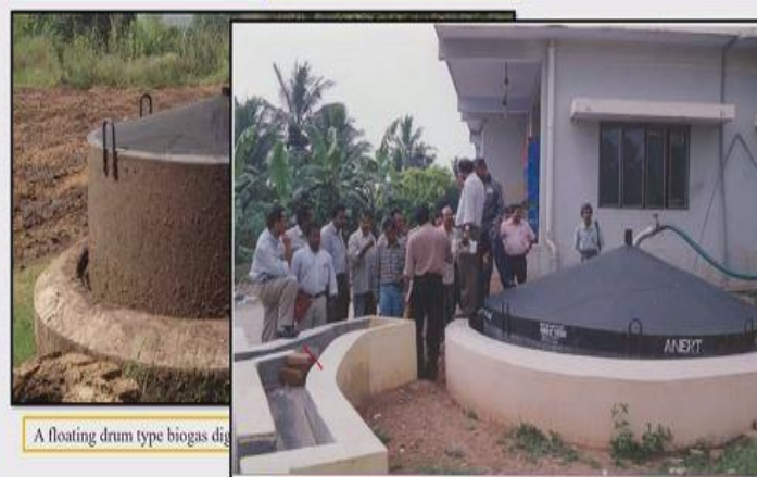
A 35 m 3 floating drum type biogas digester at Hindustan Latex, Trivandrum, India, utilizing canteen waste
