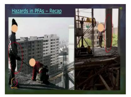
These are some of the hazards in personal fall arrest systems, for example this is not a permanent anchor. The lanyard is not anchored properly to a permanent anchor and this person is actually used as an anchor for the lanyard again these are not a proper ways of using a lanyard.
