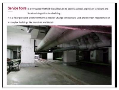
Service floors, is a very good method that allows us to address various aspects of structure and services integration in a building. It is a floor provided whenever there is a need of change in a structural grid and service requirements in a complex buildings like hospitals and hotels.
