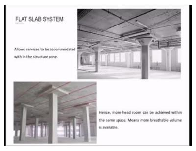
Flat slab system, allows services to be accommodated within the structure zone. Hence more head room can be achieved within the same space, means more breathable volume is available. (**Refer Slide Time: 05:29**)
