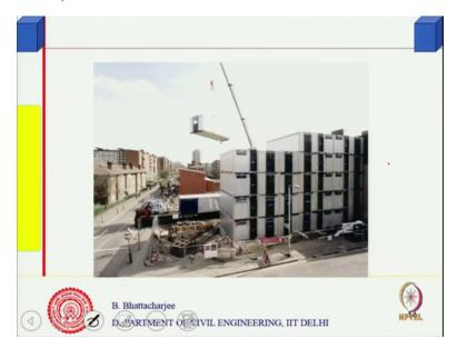
For example, this is what it shows a crane just putting the 1 module module straightway. So very useful again for similar where there are repetitive units like hostels, hotels and even apartments. So simply one can you know put them straightway the module.
