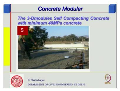
So 3D modules with self-compacting concrete obviously strength has to be high because section will be thin and it must take all handling load. Actually more crucial is the handling load, so minimum 40MPa concrete is what is required.
