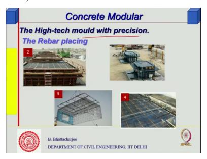
So they would possibly look something like this. There is a casting of a module casting of you know the set of so you have got number of, number of actually casting not a single bed number of casting bed, for each module there will be 1 bed, there is a kind of reinforcement, placing so then once you know the cage comes in, the whole thing comes in there is a formwork and then you do the concreting so precision is definitely required.
