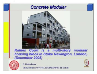
So this is what it is, so that is what. For example, concrete modular a building. This is multi-story modular housing block in London, December 2005. So this is all modular precast modular
