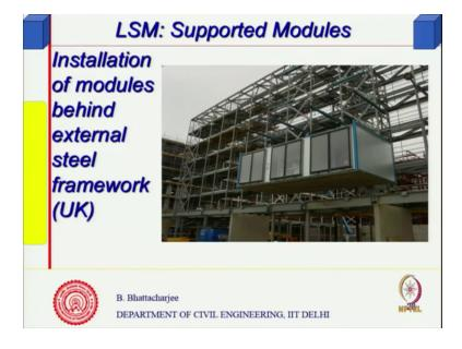
In this one the frame is there already then the modules is supported by the frame and installation of modules behind external firsts steel work has been (produ) frame you create then you put in the module.
