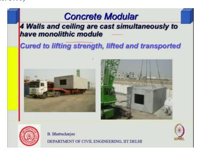
So then this is transported, whole module is being transported, lifted up and you know ceiling cast simultaneously monolithic module so everything is cast in one go, so it is monolithic even structurally it will act altogether. So structural stability from point of view it will act all altogether therefore, the performance better and you can save onto material. So cured to lifting strength minimum strength is required and then transported
