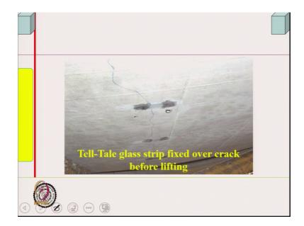
So, this example wise this was done you know this was done in this was done in that segment that I was talking about. So, this is a blue coloured crack you can see not the double red blue colour crack. And there is a glass piece you can see that being put in strip
