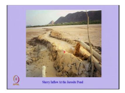
This is a process fluid coming out from ledging tailing process. So, it is slurry; it is in put in a pond. So, this is basically going to deposit it is called the Jarosite process fluid and this will impact the environment.
