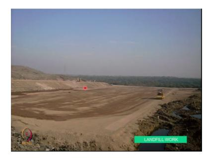
So, this is again the something waste dumping develop. That is the old waste dumping height is being raised this is the new landfill being constructed.
