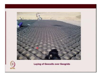
We look at it in the slope stability issue, but I just want to show you that grass in the paver blocks along the side these are Geocells, I said Geocell filled with soil; Geocells are nothing, but 6 inch high accordion arranged bands of geosynthetics.
