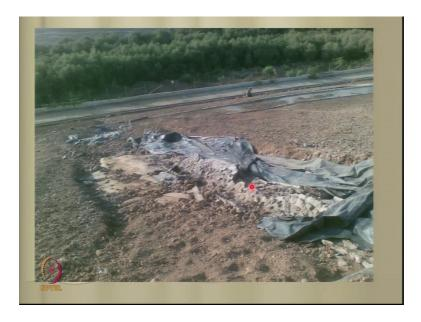
Make these layers very thin then the geomembrane can get exposed because you can slide along this. So, unless you have a good vegetative cover which is form and sustain if you make the thing very thin they are highly prone to erosion if it was thicker then at least we would have an erosion gully, but you would not have reached the level of a geomembrane.
