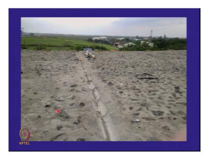
So, at the this is the green landfill grassy green this is made of rubble masonry, but the pollution control board is saying is not green and 2 two issues here this if this is settles with time they are going to be large number of cracks we can repair it no doubt about it.
