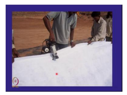
So, we have to assured it is like saying when you weld 2 steel sheets the steel joint should not leave we have to do that. So, now, I on the on the geomembrane, we are putting a protector and I am stitching this, this is nonwoven geotextile. Let me see if I can show this to you on this projector.
