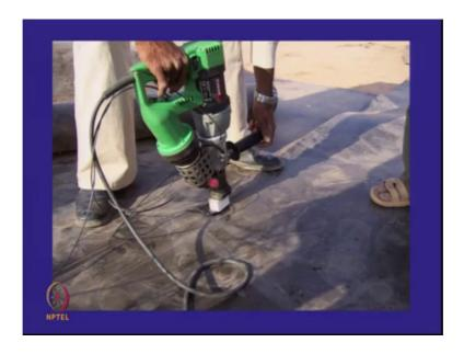
And there was a he is doing patch welding here there was a tear. So, a batch is being applied.
