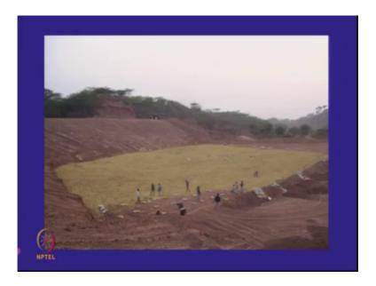
So, here you have mixed you have spread the bentonite on the soil. And you are doing what is called increase mixing you are using a tractor with plows.
