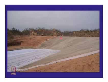
Rounded, now you can see the soil is complete and it was ready to receive the waste. So, make an impervious thick base, put a geomembrane on it, which comes out in the form of rolls and then make the other elements.
