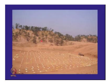
So, all this earths' work you have to cut and fill. And you are creating one phase for one year. And here you are I talked to you that if you do not have clay, then you have to mix with bentonite so that you can reduce the permeability. So, here the soil did not have 10 to the power of minus 7 centimeters per second and bentonite is available to us like cement.
