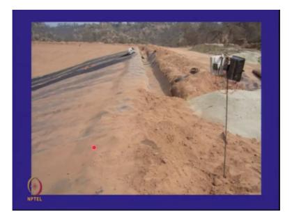
The geomembrane on the side slope and it is being anchored in an anchor trench at the top and the roll has limited width it is cut to be welded together.
