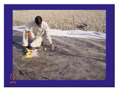
I want you to remember this. I come back to this short this is a foot pump. So, he is pumping in air in the joint. Now how he is pumping in here in the joint we will come to later there is a peculiar way this joint is made, but I can tell you whether 20 meters of this length is leaking or not. So, I make a joint it has to be a leak proof joint and in geoenvironmental engineering or environmental geotechnics, this is the most critical part. The geomembrane is fine the joint should not leak.
