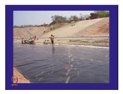
We have that is the geomembrane that is the joint. That is the nonwoven geotextile being placed over the geomembrane to protect it as a protector and geomembrane and you can see people walking over it of course, he is barefooted and you can see this white protector and on top of it you can see the leachate collection layer and this looks like sand or more.
