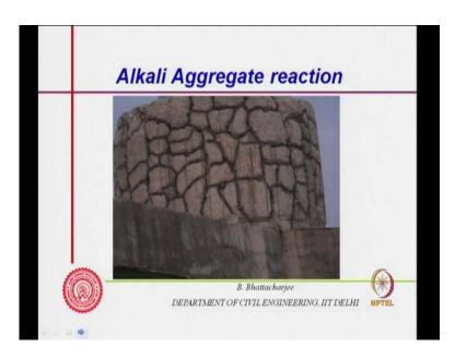
This is the real case, where the alkali aggregate reaction is caused this particular structure, you know this all source of splintering out practically, everything is going out everything is popping out. So, this is an example of alkali aggregate reaction.
