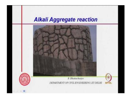
Remember this does not occur you know. So, this is the concrete complete crack in the later stages, remember this does not occur in the beginning, it takes at least 5, 10 years time. In India era could damage an example of you know it phase this problem. So, normally aggregates are tested prior to their use aggregates are tested prior to their use.
