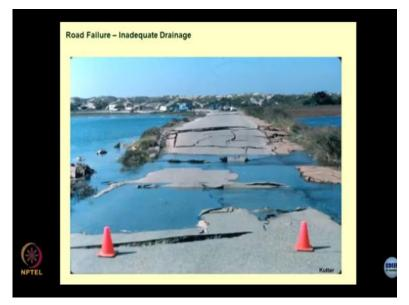
Look at this, this is the road failure, again because of the inadequate drainage, so both sides of water bodies and or the same water body and this was reclaimed, did not allow drainage to occur, water has found its own path, the road has collapsed.
