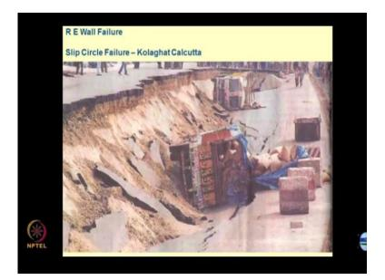
Now, this is the time of the construction of the highway. Anyway the essence of the story is that half of the road has collapsed. And these are the real life photographs, poor filled material or maybe lack of compaction or whatever, look at the whole system has cracked, the foundation failure.
