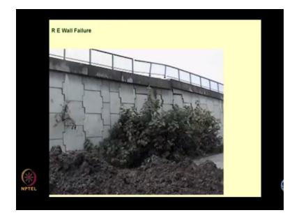
The RE wall failures, you must be reading in newspapers, there was a video also recently that the RE wall has failed somewhere. This is a good sign to see that how RE reinforced earth wall. This RE means reinforced earth wall it has failed. Look at the cracks which have developed.
