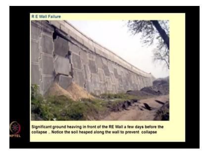
If you see from the other side of the RE wall, then you will see that how the collapse has occurred. The pile material has come out of the wall, panels have dismantled and the wall is defunct. Remember each of these projects is going to cost at least 40 50 crores. And once these type of things happen, there is no retrofitting. You cannot retrofit anything. You cannot make them overnight.
