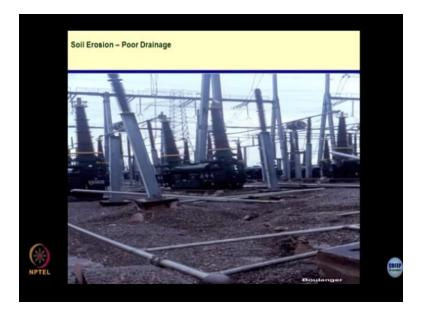
Now, look at this, this soil erosion is occurring and these are the transmission what do you call them power houses alright. So, this is where the foundations of most of the power structures are located. But because of the soil erosion, what is happening, all the structures are in a dilapidated condition. How would you deal with this type of situation, say strategy situation.
