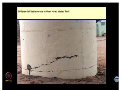
So if you have a very close view on this, you will see that the whole tank is settling on the one side, and it is cracking also from the base. Again, because of the poor soil conditions, silos, I do not know how many of you are aware of silos. Silos are the places where you store greens alright , fertilizers, granular material. So there is no difference between sands and wheat and rice and sugar. They are all granular materials for me.
