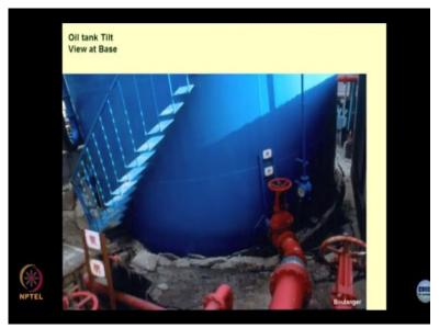
This is a very close look at what was the problem is this type of situation occurs in the tech forms, all the piping arrangements which have been done at the funk, they have cracked why, because you are designed these pipelines to be connected to a certain portion of the tank. When the tank settles, so these pipelines have got sheared off or veered off or they have got cracked completely.
