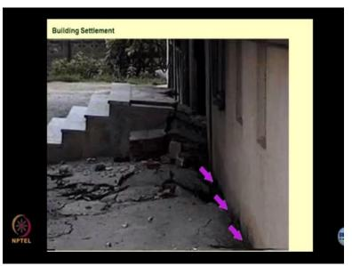
There is another good example of how building settles, I was talking about when we were discussing, the staircase has completely got detached from the building. The plant has cracked, the building is going in, as a matter of few days when this will be in the national network.
