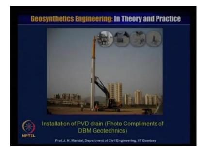
So, here you can see that installation of the prefabricated vertical drain, this is photo compliment to DBM Geotechnics. And this is the only, this one rig and this is very soft soil, where the prefabricated particle drain has been installed.
