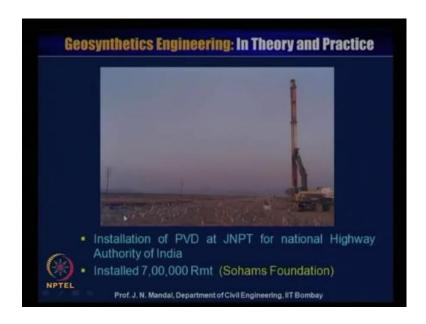
So, you can see more the installation of PVD at JNPT for national highway authority of India. And this is all white color here, this is prefabricated vertical drain has been installed. And this install about 7,00,000 running meter, this is Sohams foundation.
