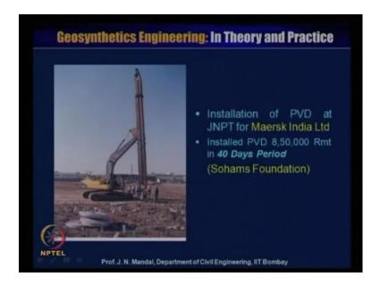
Here is also installation of the prefabricated vertical drain, you can see this is the, in the roll form like a roll of used toilet paper. So, this is the prefabricated particle with this crane, this prefabricated vertical drain inserted to the desired depth and then on the, from the top you can cut it, with the help of a scissors. So, this is the installation of PVD at
