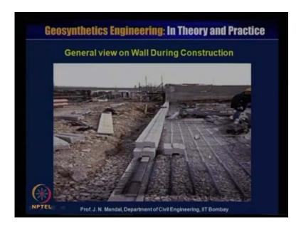
You can see how this geo grid material has been replaced and how, it is connected how the block is placed, this is a general view of wall during the construction.
