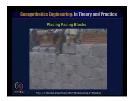
You can see how the placing of the facing blocks, one with the other you have to place the properly, the lift should be proper it should be joint, it should be connected the geo grid material with the block in proper placing.
