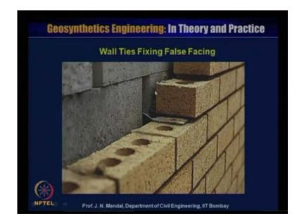
You can see wall ties existing the mobile with the false facing element here.
