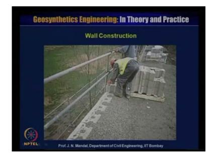
And you can see the wall how it is constructing and this is h filled up, with the aggregate it will act as a drainage, this is the block, so it is in the small mall block and the weight is not, so much. So, one can carry and can fix it up and then you filed up with the aggregate for the drainage.
