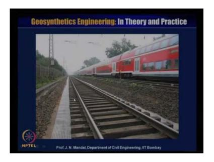
You can see you can place the geo synthetics material here and then mud pumping can be controlled also.
