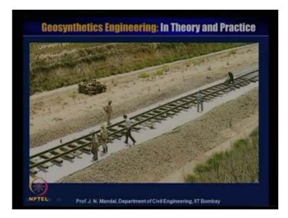
You can see here that, how the geo synthetics material this white color has been used this below the this railway track.
