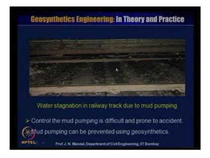
So, water you can see here water stagnation in the railway track due to the mud pumping., so you need control the mud pumping is difficult and prone to accident mud pumping can be prevented using the geo synthetics material.
