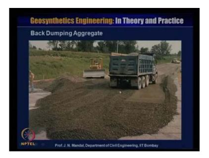
So, this is the back dump of the aggregate, you are back dumping this aggregate, aggregate is inside the truck you are back dumping this aggregate.
