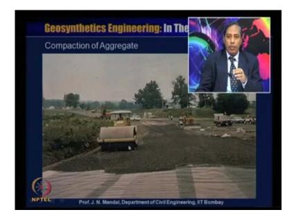
You can see how the compaction of the aggregate by the smooth roller, how it is compacting.
