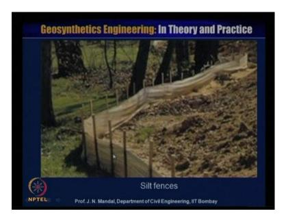
So, this is silt fence which is preventing the precipitation run off under flow. So, you can one of the silt fences here, how it has been precipitated.
