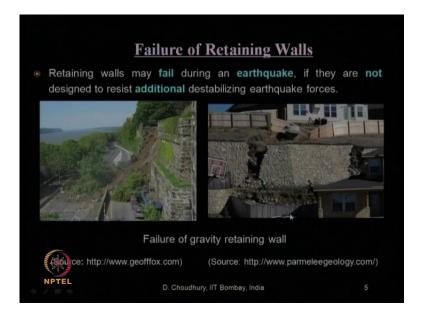
Same remains in the case of earthquake condition also. There are various examples worldwide – the failures of retaining wall due to the additional destabilizing earthquake forces, which comes on the retaining wall during the earthquake process. So, unless we estimate this extra or additional destabilizing earthquake forces on the retaining wall and consider those for the design of retaining wall, then failure cannot be avoided.
