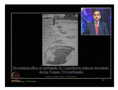
This is another picture, which shows the devastating effect of earthquake by liquefaction induced movement. So, after the liquefaction, the soil or watery soil – I should mention –
