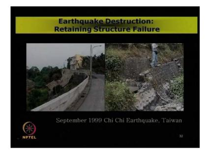
Coming to other form of earthquake destruction like retaining structure failure or retaining wall failure, this is the initial retaining wall. You can see one portion of it got collapsed over here after the 1999 Chi Chi earthquake in Taiwan. This is the close view of that collapse of that retaining structure or retaining wall after that earthquake.
