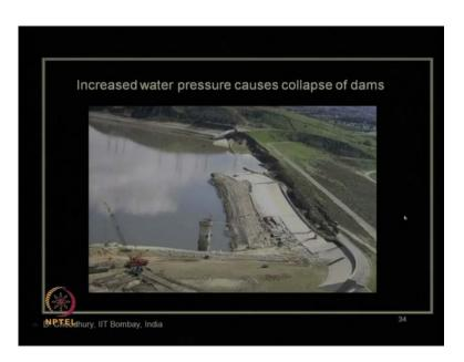
Another picture shows here the increased water pressure, which causes collapse of the dam. You can see over here at this portion, the dam has been totally collapsed. This is due to the increase water pressure during the earthquake condition.
