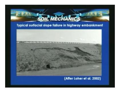
So what happened is that this unstable portion was detained by driving recycled plastic pins into the slope so the cross section is shown and the failed area so entire area is actually strengthened to prevent this slope.
