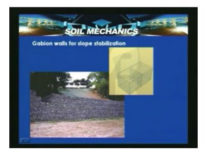
Another method is the gabion walls for slope stabilization. In this technique what is done is that this gabion walls are nothing but is wide measures which are pre dominantly made with mild steel which are coated with anti-corrosive elements. So in this if the area is actually having abundant availability of stone, the stone is actually filled in this cases and placed one above the other and with that actually these types of walls can come.
