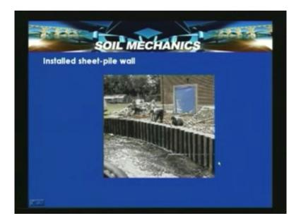
So these are also being in flexible in nature they are also called flexible retaining structures. So from here onwards we are trying to look into different types of flexible retaining structures and how these flexible retaining structures can be analyzed, what are the salient aspects in the design that we look into it.
