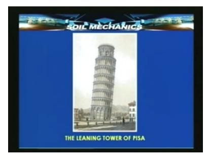
What is special about this is, one side of this PISA tower has undergone settlement due to a compressible soil layer below it and this has recently been rectified and it has been ensured that it will remain tilted and stable at a particular degree of rotation. Now why did it settled? Let us understand. In the first case some details the subsidence due to the clay layer below is 1.89 meters that means one side of the tower tilted by 1.89 meters.
