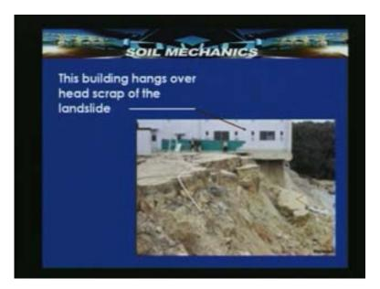
This particular building as you have seen in the figure shown above is hanging on the top of the landslide debris. And these sort of things really causes alarming signals for the soil mechanics engineers.
