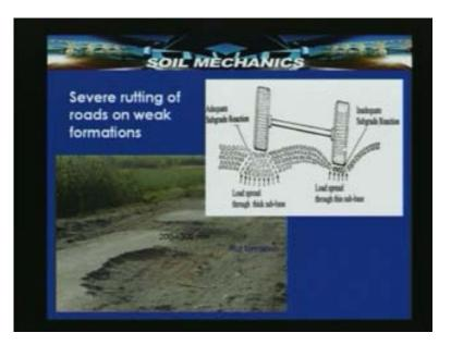
This particular case history shows a severe rutting of roads on weak formations. So this can create a rutting which as shown which affects the ride ability of roads.
