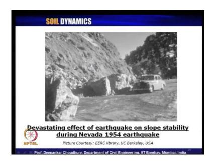
Another picture, which is again taken from EERC library of U C Berkeley, it shows the devastating effect of earthquake on the slope. That is on stability of the slope during Nevada 1954 earthquake. The land slide or slope stability problem arised and all the failures have taken place for the slope, due to the earthquake loading. So, that again needs the knowledge of the soil mechanics and the rock mechanics etc to understand the behavior of these material under the dynamic loading.
