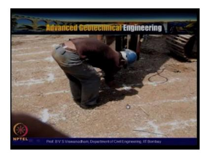
So we will actually look in to the installation how it actually happens in the field, so here you can see the softness of the clay the this is nothing but is the drainage blanket and the mandrel is actually being driven in to the mandrel is being driven in to the ground. So this is the vary house corporation which is actually existing given house corporation and this is also for you know enabling in a placement of the loads over that area.
