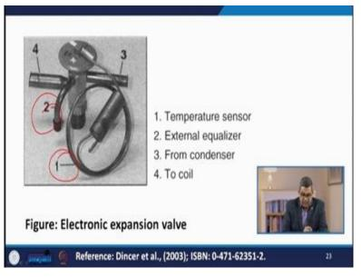
Now here you see that this is the electronic expansion valve. Now here this is the temperature sensor and this is the external equalizer. This is the inlet line from the condenser and this particular line goes to the coil.
