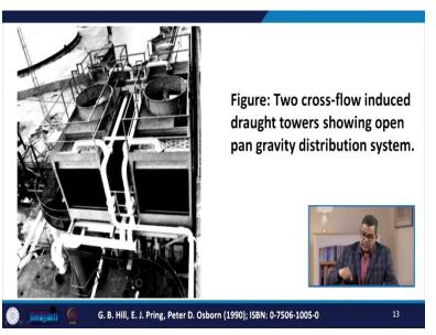
Here you see that this is the two cross flow induced draught tower. This is showing the open pan gravity distribution system.
