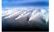
Here it is mentioned that a simple rule of thumb the turbines follow the spacing rule of 4 rotor diameters apart horizontally and 7 rotor diameters apart vertically in the wind's direction. So we have made some discussions on wind energy productions. Thank you for your patience.
