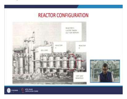
Now you can have a more closer look of this a particular reactor battery. So these were the 6 reactor and this was the off gas manifold and this was a problematic reactor.
