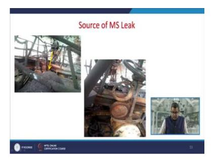
Now, this was the source of motor spirit leak, now you can visualise there are hand operated valve motor operated valve and this one is the blind, blank, now this is the mean scenario so it was not been inserted properly while the transfer took place.
