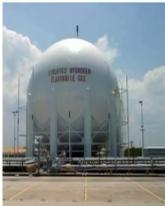
Storage tank at NASA, 3800m<sup>3</sup>, 270t, 21 m outer dia, 6.2 bar, 0.06% evaporation rate
