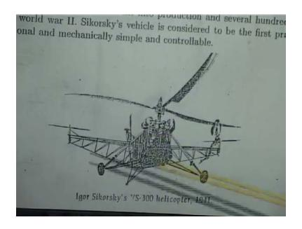
See, here in this picture you will see, there is one rotor here, one rotor here, there is one rotor here and then one main. These are two horizontal thing, initially this model had this, later he removed these two horizontal rotors, put them in the middle as one rotor, later that also he removed.
