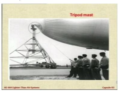
I want you to look at various types of mooring masts. For example, this is the tripod mast. A large tripod mast which is nothing but like a camera tripod. In this case we have wheels so that
